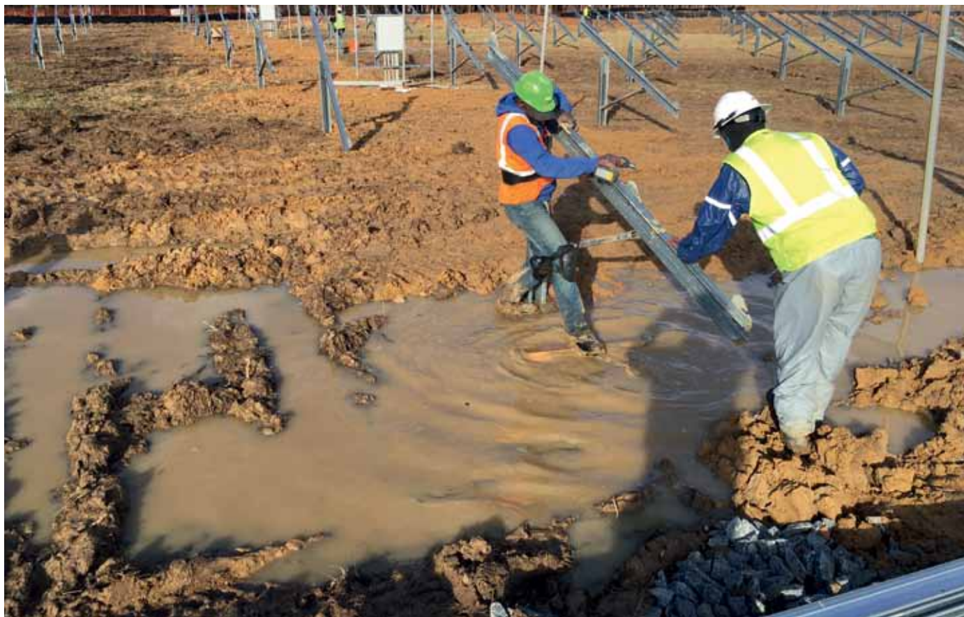
Pressures arising from the U.S. tax calendar have sometimes forced installers to work in poor conditions. This can lead have an adverse effect on the final quality of an installation.
